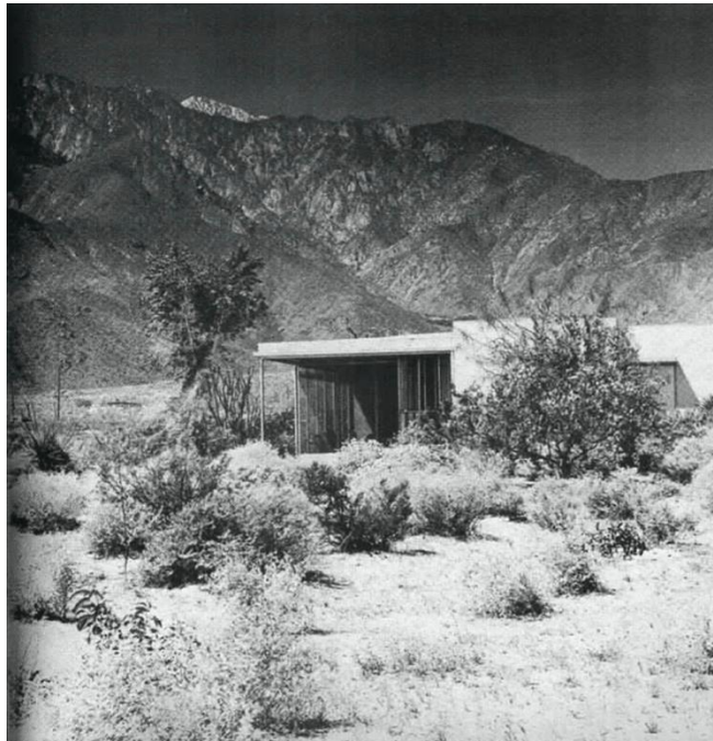
Figure 13. Miller/Mensendieck House, 1937. (Photograph in California Arts and Architecture , May 1937.)
