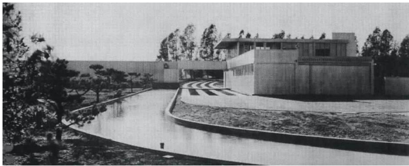
Figure 10. Exterior of the Von Sternberg House, 1935.
