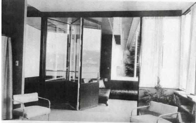
Figure 5. Folding doors between living room and sleeping porch, VDL House, 1932.
