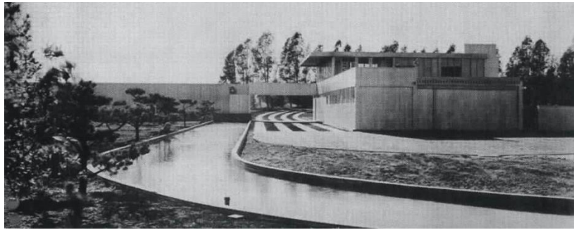
Figure 10. Exterior of the Von Sternberg House, 1935. (Photograph by Yukio Futagawa.)
