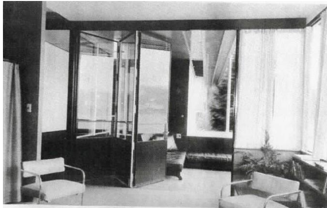
Figure 5. Folding doors between living room and sleeping porch, VDL House. (Photograph in Architectural Forum , November 1934.)
